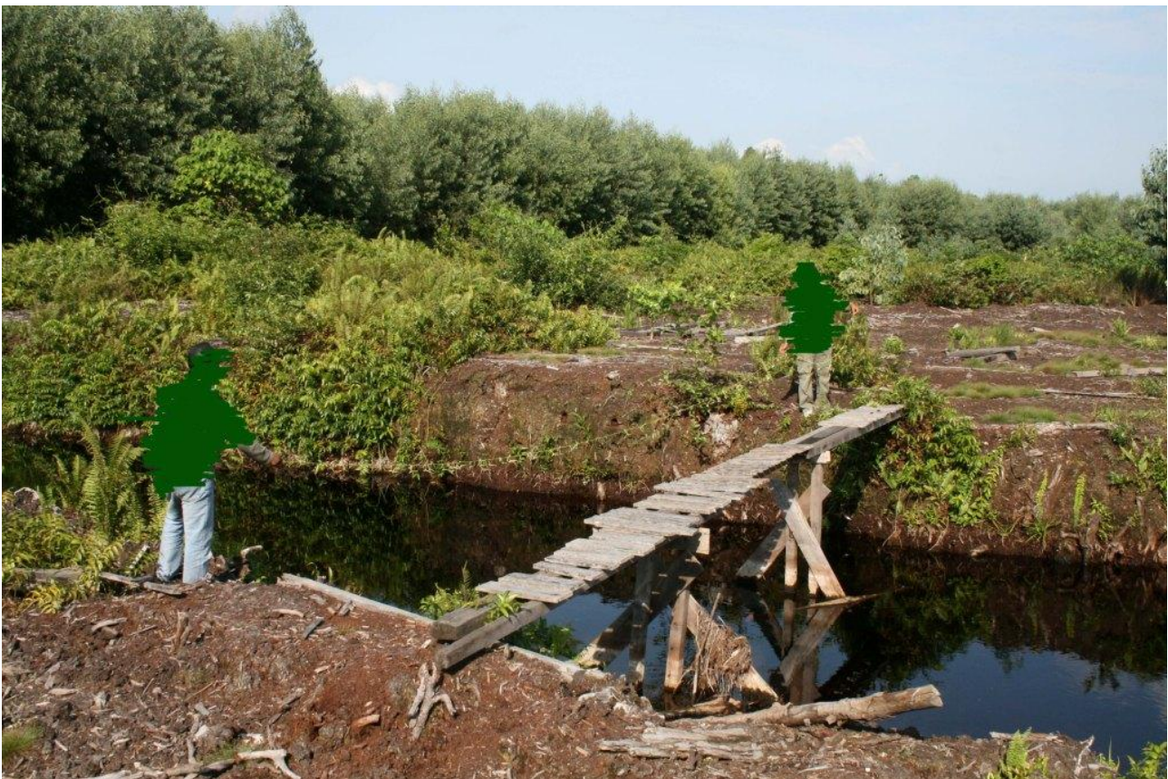
Photo 3. Canal next to the APP logging highway at (GPS location 2 in Map 4). In this location, water surface was about 2 meters below the top of the bank.
