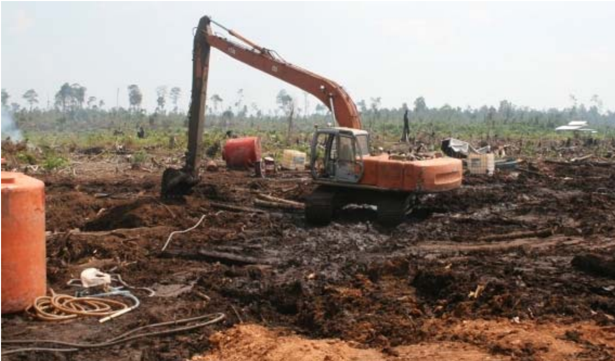
Photo 2. An excavator of PT Sumatera Riang Lestari is digging canal in Kerumutan peat swamp forest.
